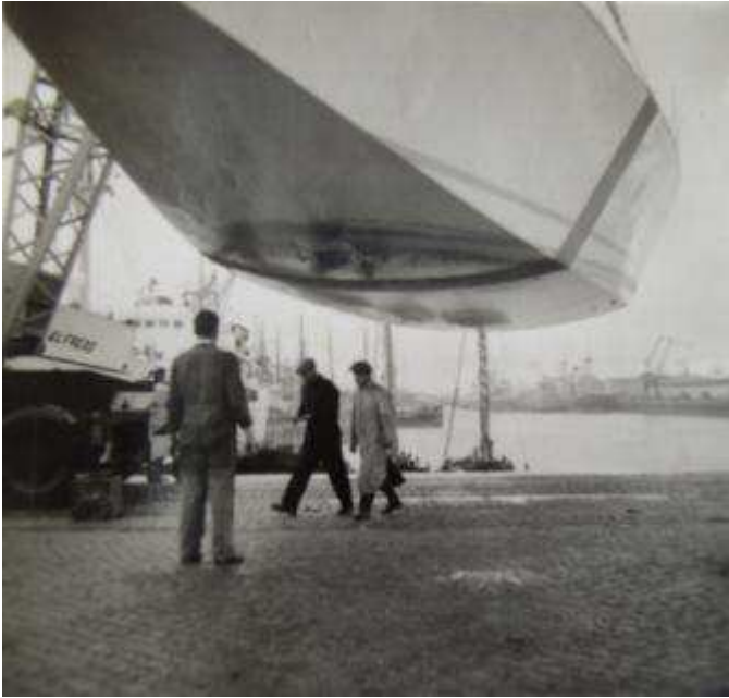
A view of the bottom before the keel, rudder and skeg were attached
